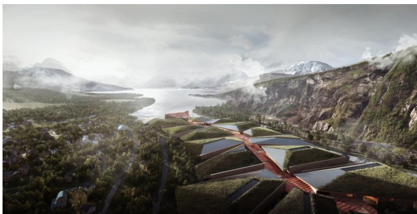
Fig. 16: This artist rendering of the Kolos data center in Ballangen, Norway - ostensibly the world's largest data center - was featured in an August 2017 press release (image from the Canadian Architecture Firm HDR, reproduced under Fair Use Licence).
