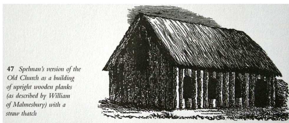
Figure 1: The Vetusta Ecclesia, as envisaged by Henry Spelman in the mid-seventeenth century, as a building of upright wooden planks (as described by William of Malmesbury) with a straw thatch (Rahtz, 2003, p.94).
